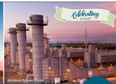
Almond Power Plant
