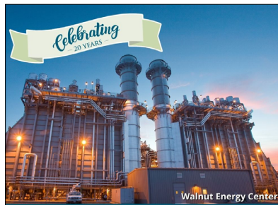
Walnut Energy Center
