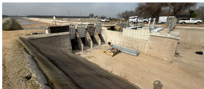
Construction progress on the Main Canal
