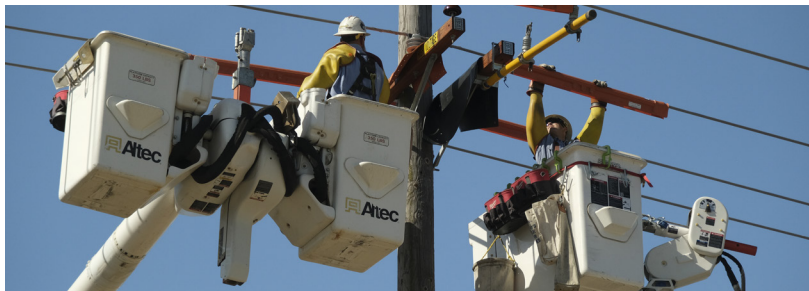
TID lineman performing a crossarm change
