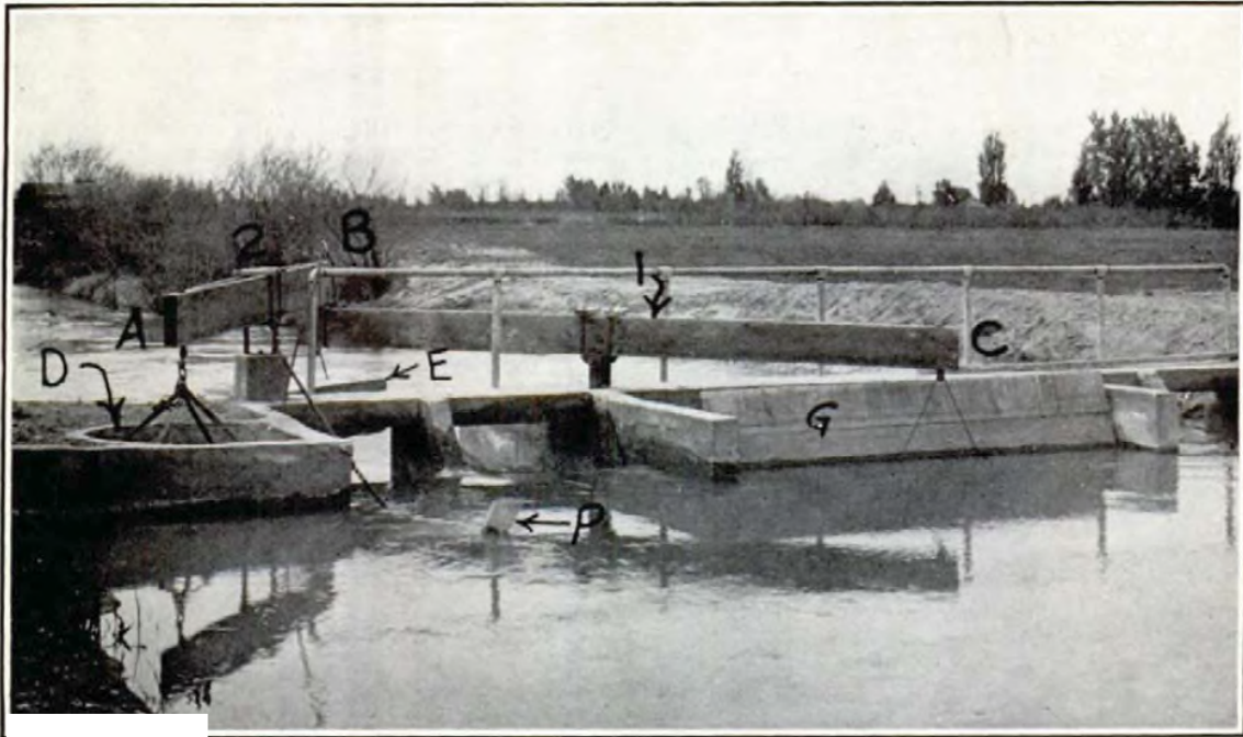
FIG. 1.—AUTOMATIC CHECK GATE, TURLOCK IRRIGATION DISTRICT, CALIFORNIA.
