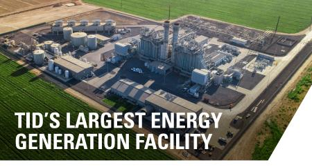
Since it began commercial operation in 2006, Walnut Energy Center (WEC) has proven to be an efficient, environmentally responsible source of reliable electrical energy serving the growing energy demands within TID's service area. Capable of generating 250 megawatts at any given time, WEC is the single largest power generation facility owned by TID.
