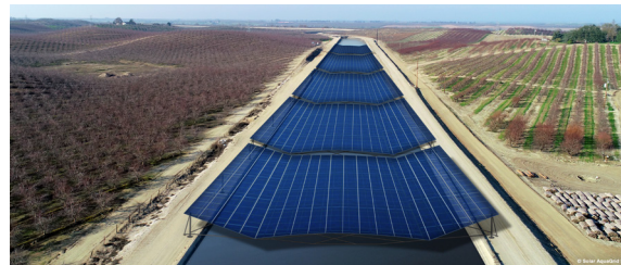
First in the nation innovation: Project Nexus – Solar Over Canals Pilot Project
