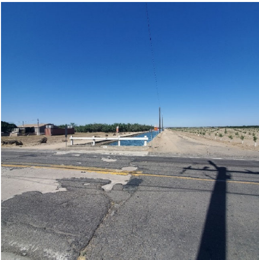
Photo 2: Upper Lateral 3 canal facing west from Faith Home Road.
