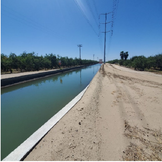
Photo 1: Ceres Main Canal facing south from E Keyes Road.
