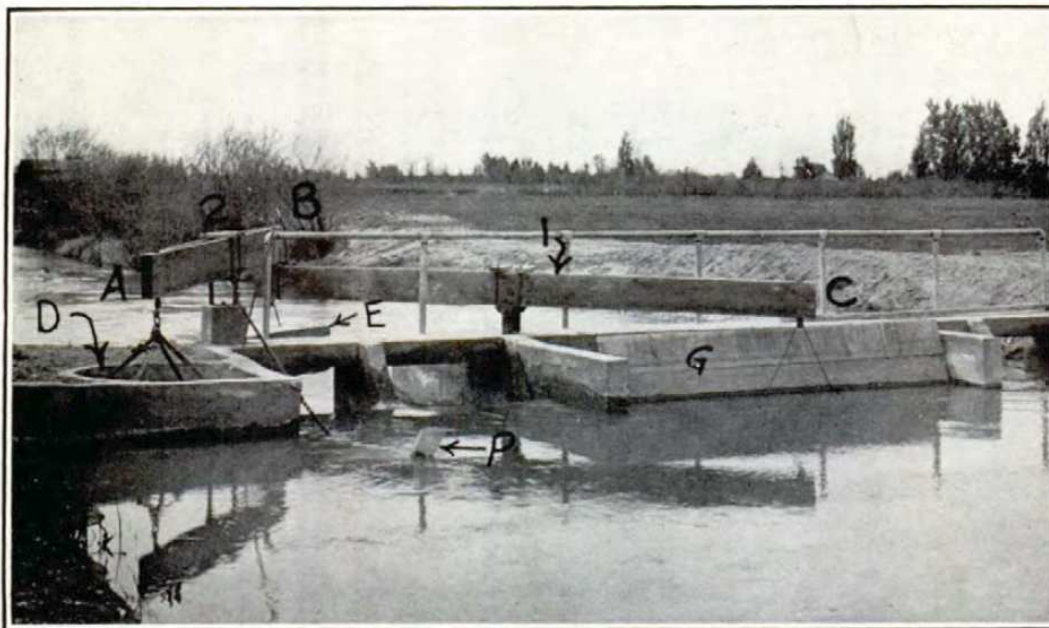
-AUTOMATIC CHECK GATE, TURLOCK IRRIGATION DISTRICT, CALIFORNIA.
